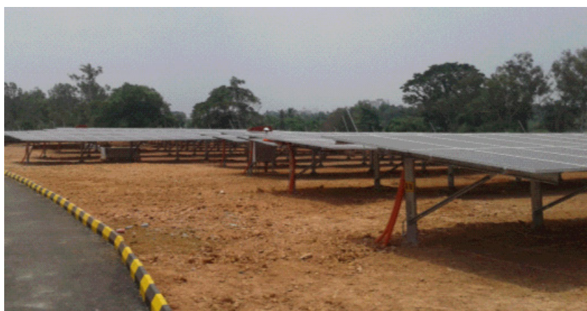
Figure 8. Solar PV Power Plant of 1.15 MW capacity at Alupuram, Kerala.
