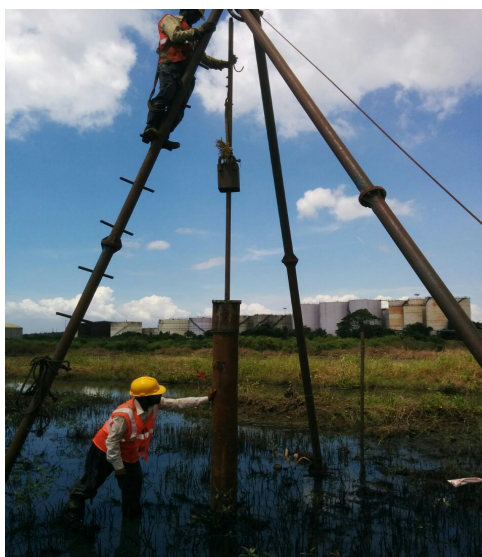
Figure 10. Pilot trials for marine clay reclamation at sea port, Mumbai.
